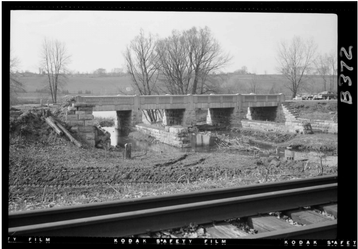
Sample 10. Canal Society of New York State Gayer negative B372, showing the Erie Canal's 1849 Tokken Creek Aqueduct near Fultonville, NY, April 26, 1953. Gayer is standing on the tracks of the West Shore Railroad. Abandoned in the 1960s, the railbed is now part of the New York State Canal Corporation's Canalway Trail. He is documenting the remains of the aqueduct. He knew that within a few days it would be demolished for the construction of the New York State Thruway. Gayer followed the Thruway's construction throughout the Mohawk Valley, recording the only comprehensive documentation of historic canal structures lost by that work. The 1918 Erie Barge Canal is beyond the aqueduct, in the Mohawk River. With the completion of that 1918 canal, the Tokken Aqueduct was reused as a highway bridge.
