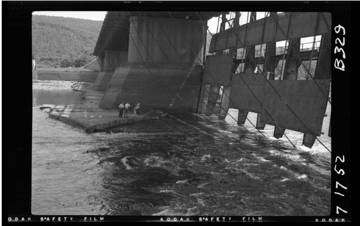
Sample 8. Canal Society of New York State Gayer negative B329, showing the dam at Erie Barge Canal Lock 9, Pattersonville, NY, July 17, 1952. The "Mohawk" dam with its moveable gates remains a classic design of the 1918 Erie Barge Canal. The gates are lowered to create a navigable depth and removed come winter. In the spring of 1952 the foundation to this dam was undermined by the fast moving waters of the Mohawk River, one the first and few failures of this type of structure. Gayer recognized that during the emergency repairs portions of the dam not normally visible would be accessible. He followed the repairs photographically until completion. Gayer was a regular visitor to structures along the Erie Barge Canal, whenever possible documenting their operation and maintenance.
